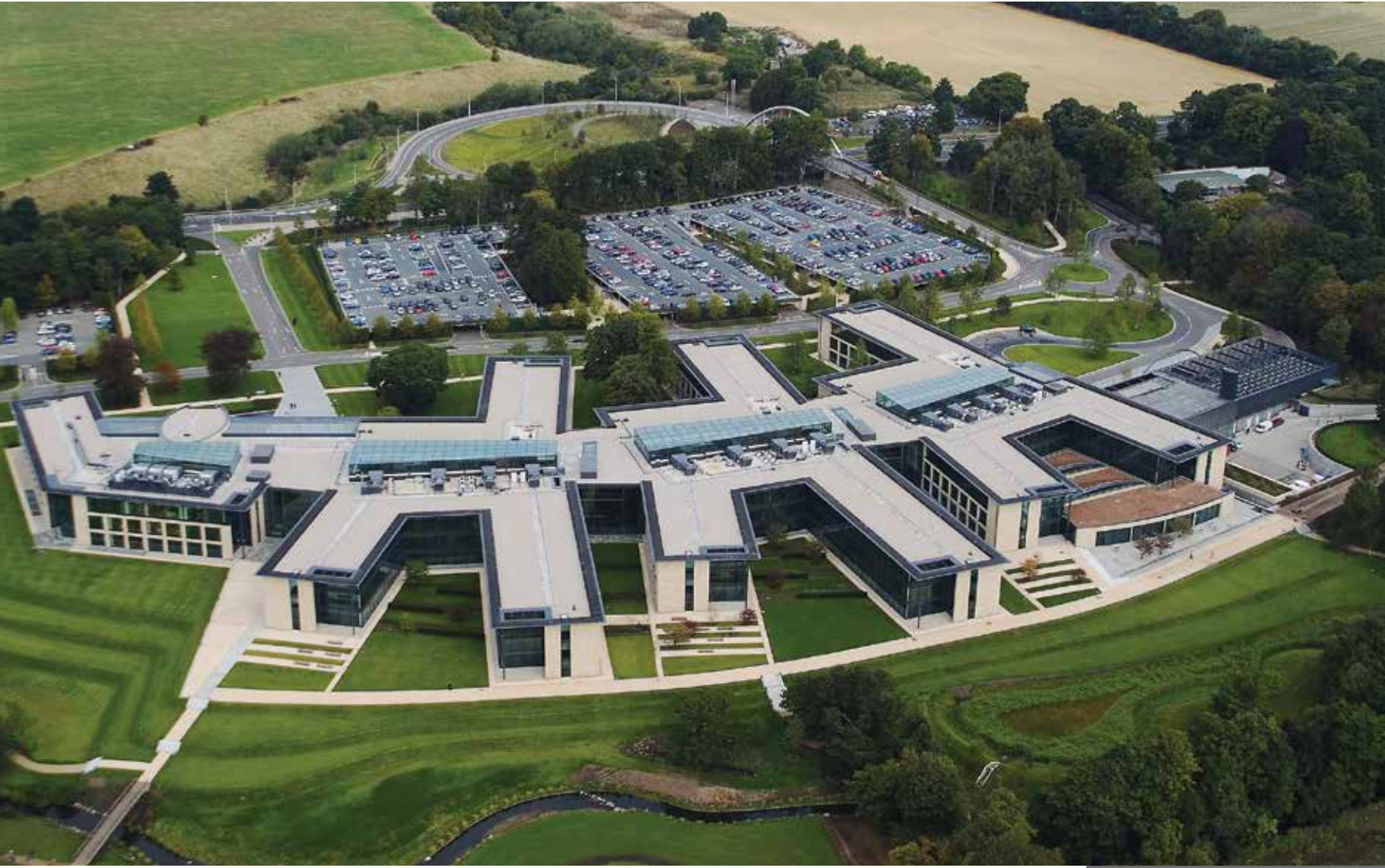
Royal Bank of Scotland HQ 2004 Edinburgh, Scotland ▲ Architect: RHWL Architects
