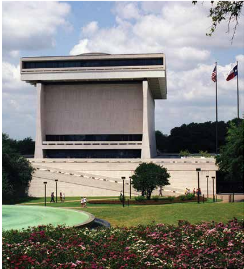
Lyndon B. Johnson Library - Renovation
