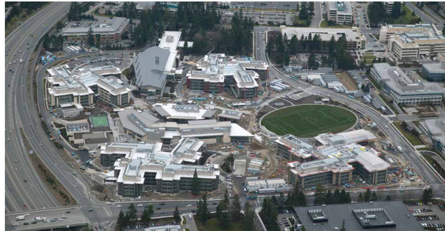
Microsoft West Campus G-98 Underground Parking Garage
