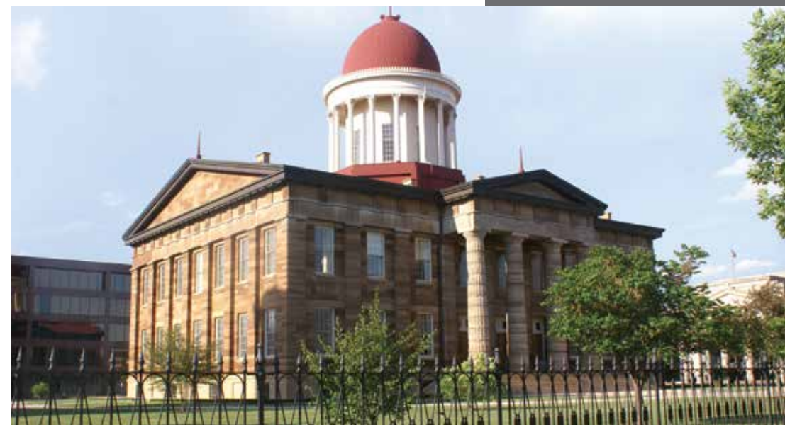
Old State Capitol - Renovation
