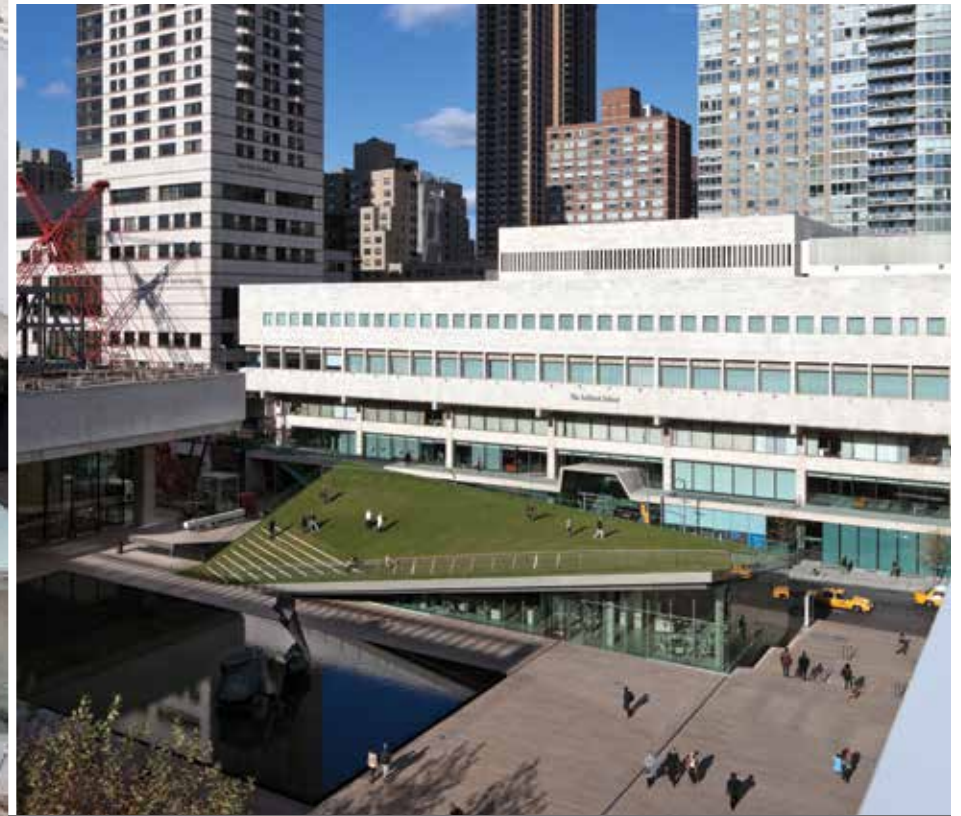
Hypar Pavilion Lawn & Restaurant located at Lincoln Center - New York, NY
