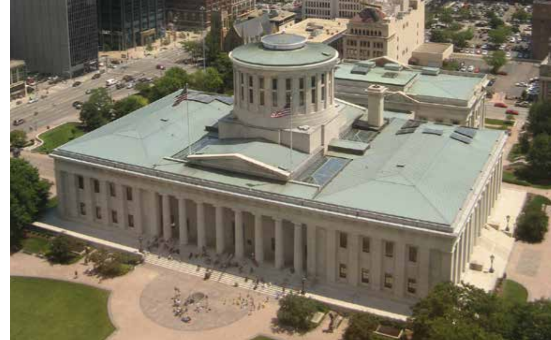
Ohio Statehouse - Renovation
