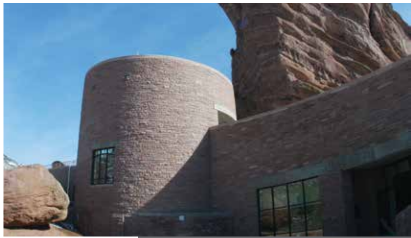
2002 Morrison, CO Architect: Sink Combs Dethlefs
