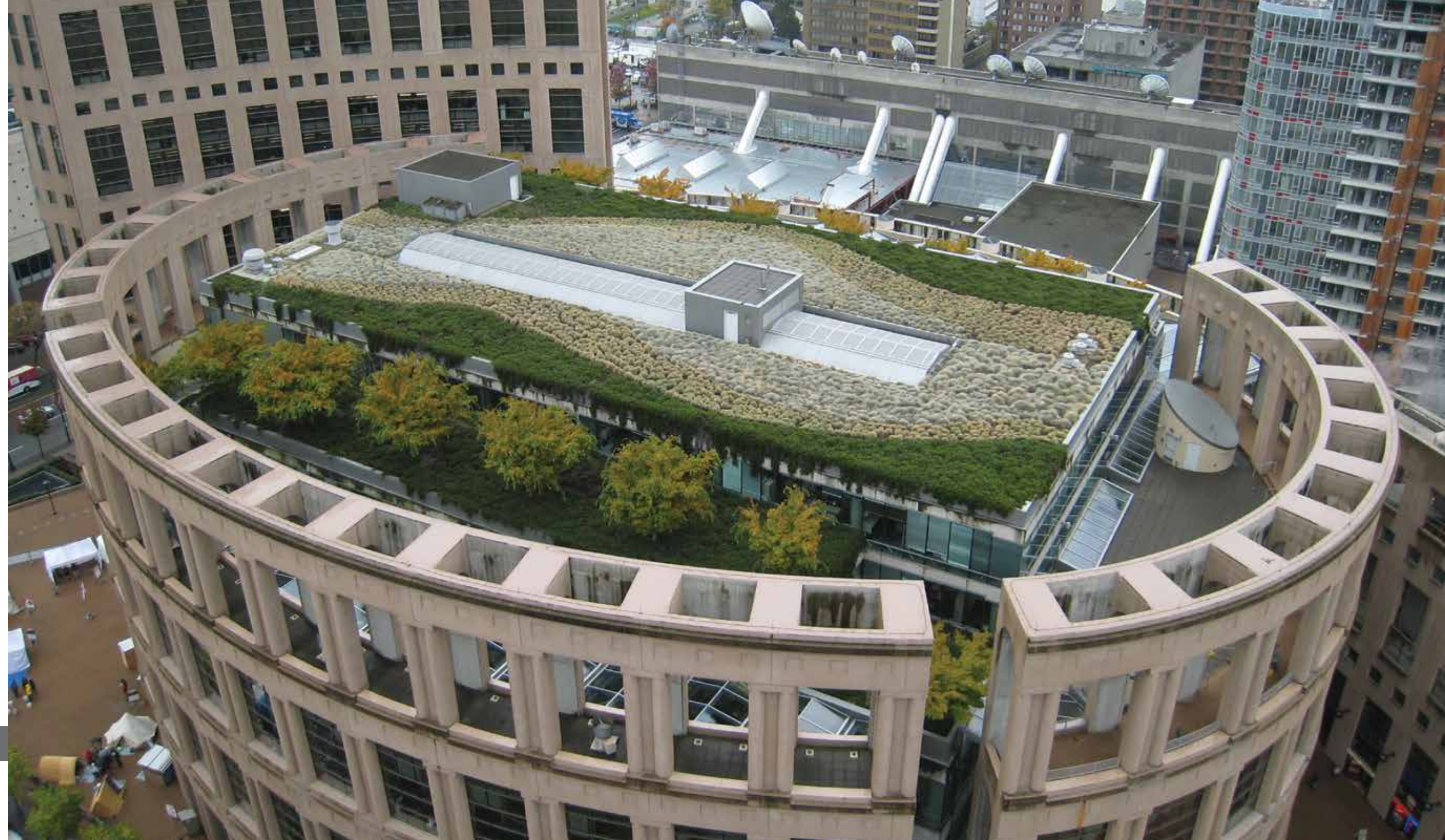
Vancouver Public Library - Central Branch
